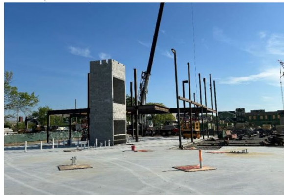
4/30/2025 - Start Erection - Area A
