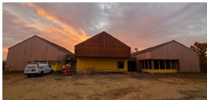
Completed façade, December 2023
