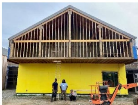
Trainees working on the façade
