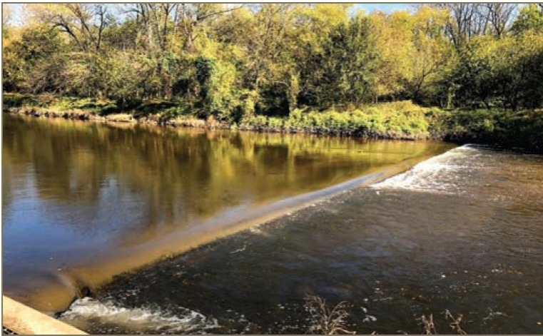
An inflatable dam helps to control salinity near the intake of SUEZ Water Delaware.
